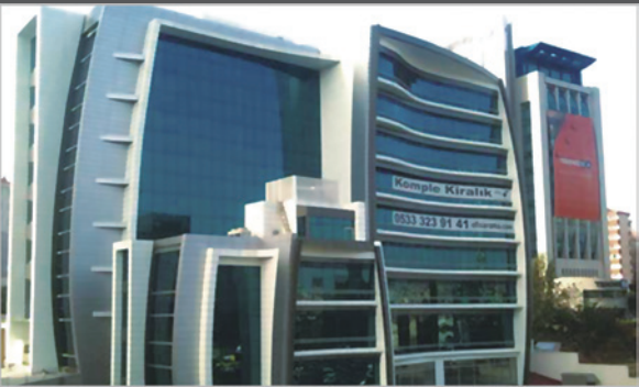
Office building in Istanbul,Turkey.
