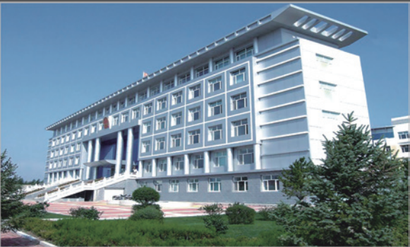
Government building in Inner Mongolia, China.
